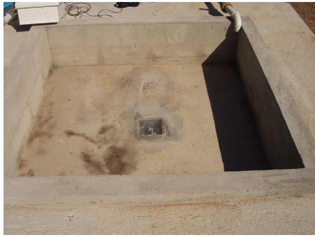
Figure 1. Solar disinfection unit.
